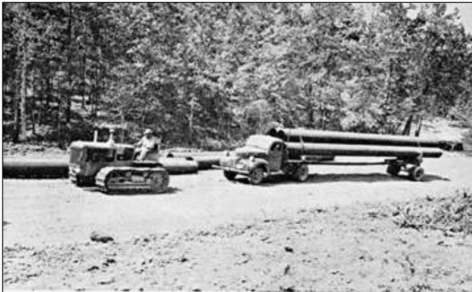
To get loads of pipe up steep hills and through mud, tractors were used, as here in east Texas. *The Oil Weekly* (6 Nov. 1944), 64 (Courtesy Gary Cheatham).
