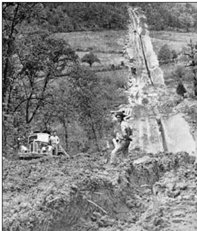
Mud a foot or more deep hampered construction; trucks were sometimes anchored to trees to provide maximum power without shifting position. *The Oil Weekly* (6 Nov. 1944), 64 (Courtesy Gary Cheatham).
